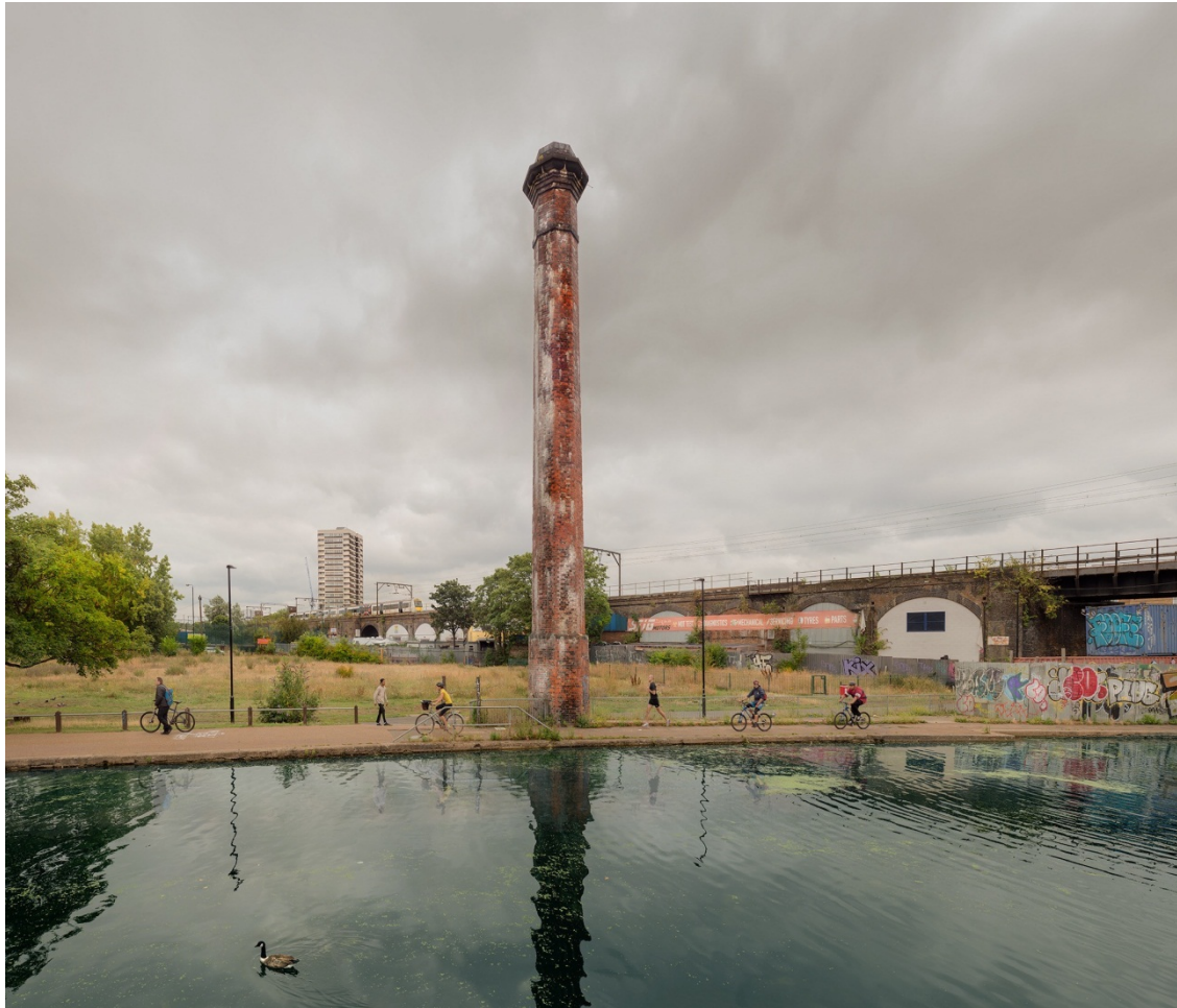
Brick Chimney in Kirk's Place
